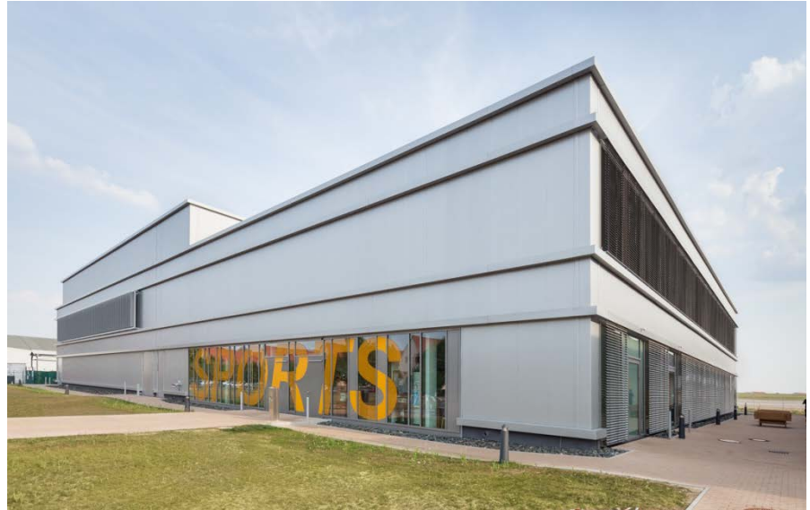
Ansicht Nordfassade Physical Fitness Facility, Katterbach (Copyright: IB Wolfrum)
